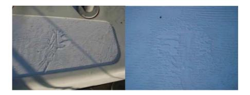
c) Position one edge correctly, and unroll the TBS covering following the furrows made by the scraper, while removing the air as you are laying it.
