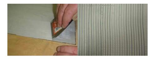
Tip: scrape the excess single-component polyurethane adhesive (figure 1) both ways (figure 2). Also scrape towards yourself (figure 3) with the scraper, giving it an open angle of 130°, depending on the support.
