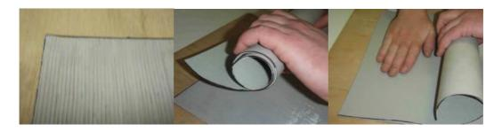
d) With single-component polyurethane adhesive, type Sikaflex 291, you can reposition your sheet during 2 minutes.
