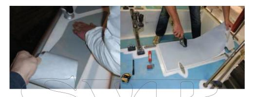
f) The laying of the TBS non slip covering is finished. The maximum characteristics of adhesive hold will be obtained after 72 hours. However, you can walk on the support immediately.
