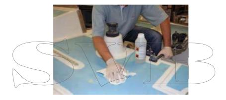
b) Using a corrugated scraper n° 0, put less than 170g/m² of single-component polyurethane adhesive, type Sikaflex 291, on the support. If you put too much adhesive, there may be waves and bubbles when you try to evacuate the air trapped under the covering.
