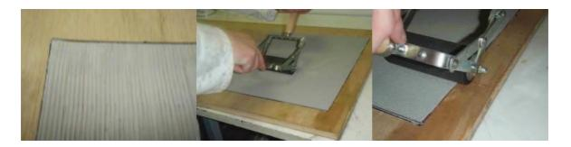
If there are air bubbles, remove them with the hypodermic needle of a syringe before the adhesive hardens (less than an hour). Do not use a cutter.
