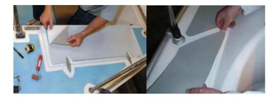
e) Once the TBS non slip covering is laid, make a firm and steady pressure one way and the other with a two-handle roll, insisting on the edges. The adhesive is pressure-sensitive and its mechanical gluing value depends on the pressure made in the beginning.
