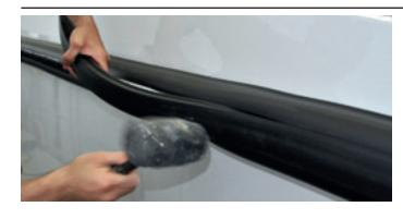
Apply the closing profile by pressing with a rubber hammer.
