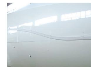
*TIP: warming up the profile base will simplify the procedure. This can be obtained by keeping the base in a warm environment for 8-12 hours.*
